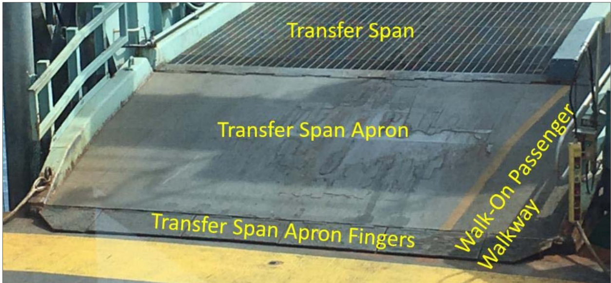
Figure 1 Transfer span components (Ref 2)
